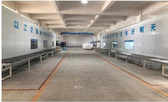
Air Conditioner Plant View
