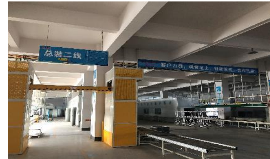
Air Conditioner Plant View
