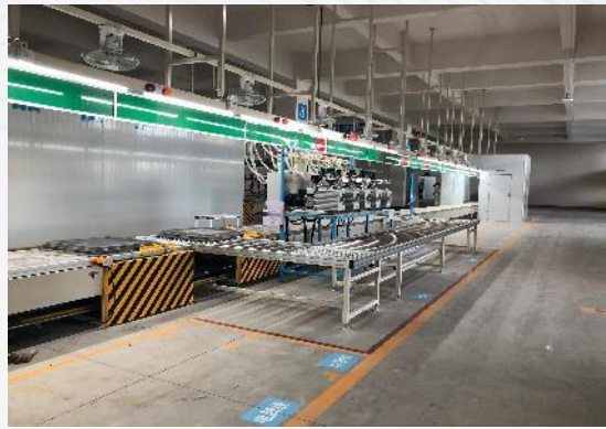
Air Conditioner Plant View
