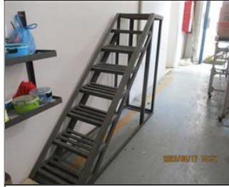
Photo of non-conformity Staircase missing handrail.JPG
