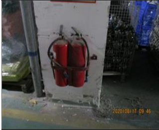
Photo of fire safety equipment Extinguishers.JPG
