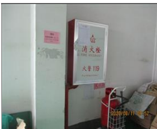
Photo of fire safety equipment Fire hydrant.JPG
