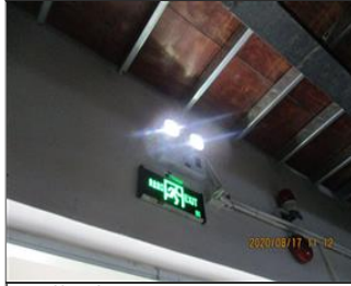
Photo of fire safety equipment Emergency light.JPG
