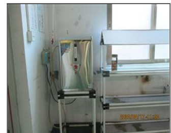
Photo of the sanitary facilities Potable water.JPG
