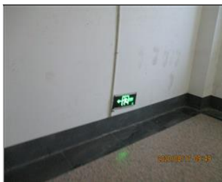
Photo of fire safety equipment Evacuation sign.JPG
